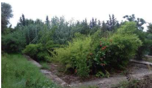
Fig 1 : Treatment plant for Jougar village
